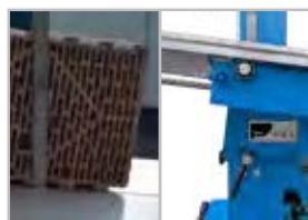
Inclined cut on bricks with empty cavities
